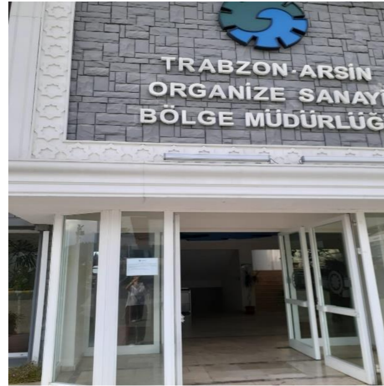
Arsin OIZ Regional Directorate Administrative Building
