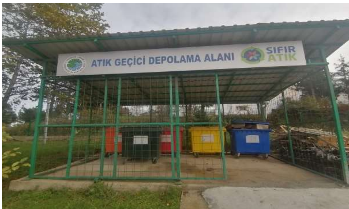
Photograph 19. Non-hazardous Waste Storage Area
