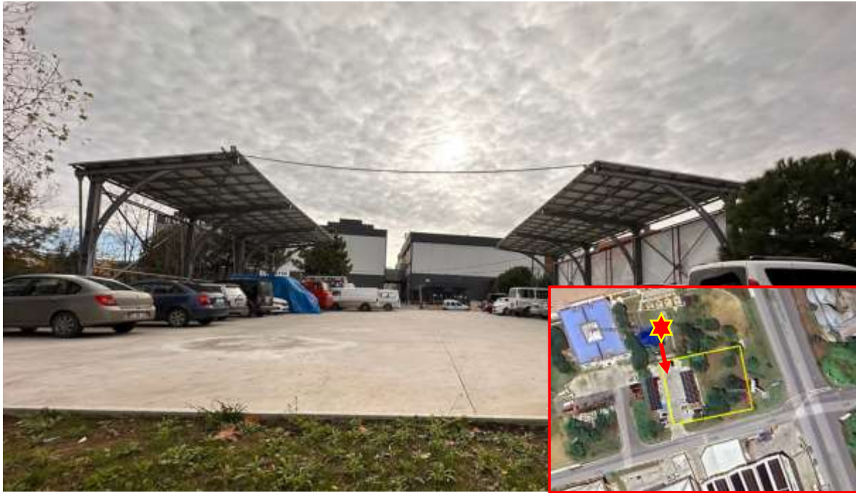
Photograph 4. Views from the Carport SPP Area-II
