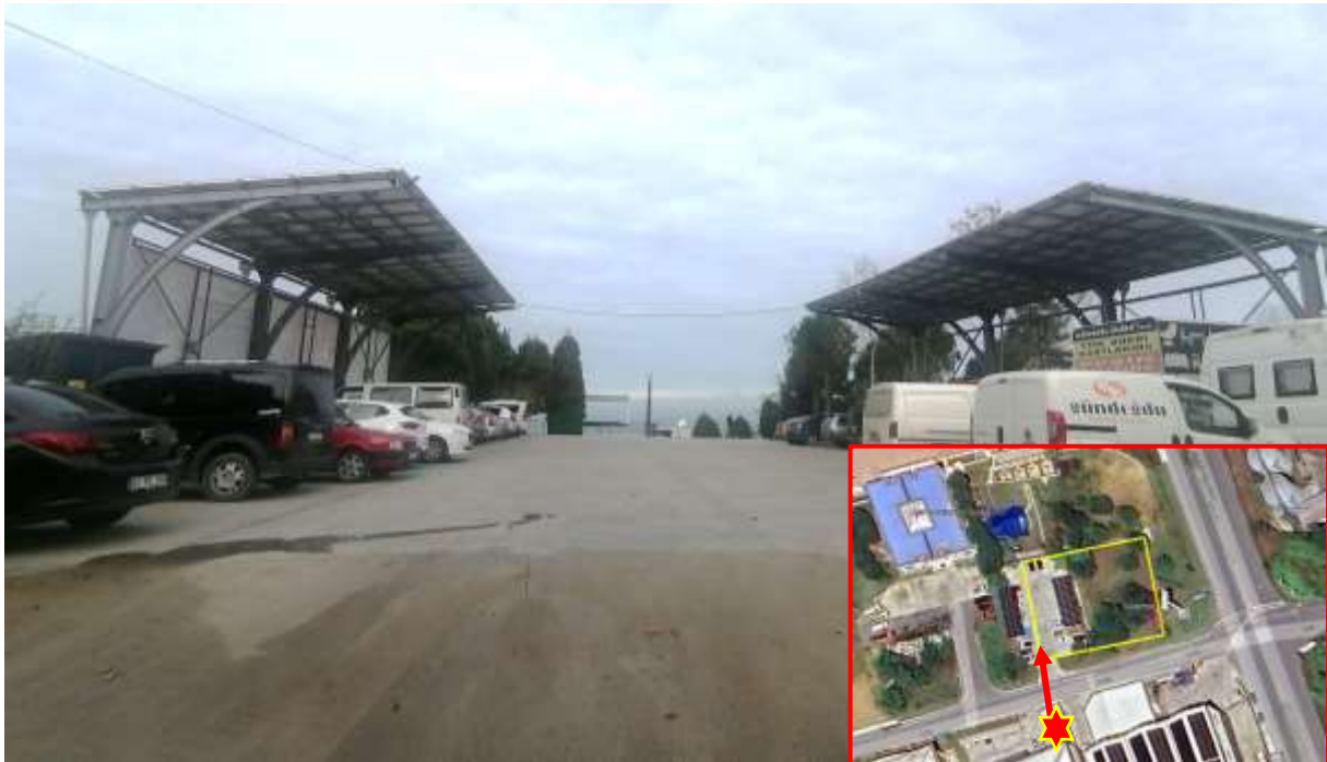
Photograph 3. Views from the Carport SPP Area-I
