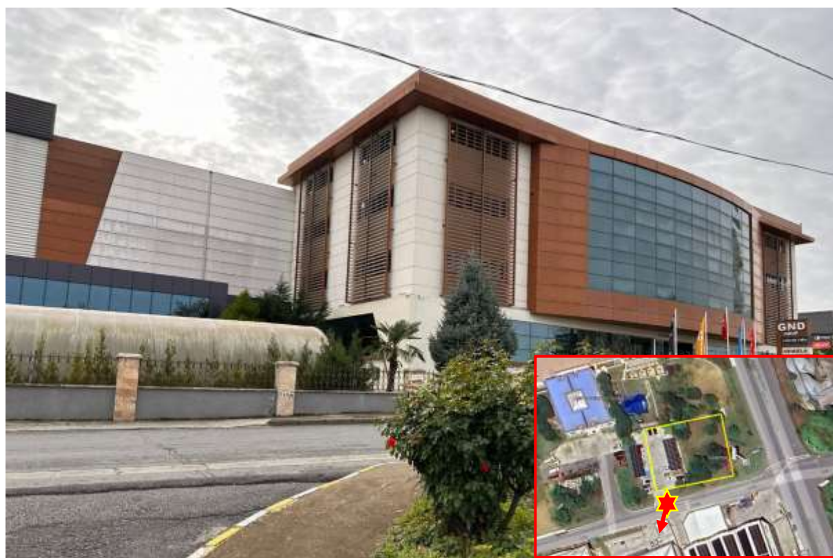
Photograph 10. View to the “Gündoğdu Mobilya” Office Building
