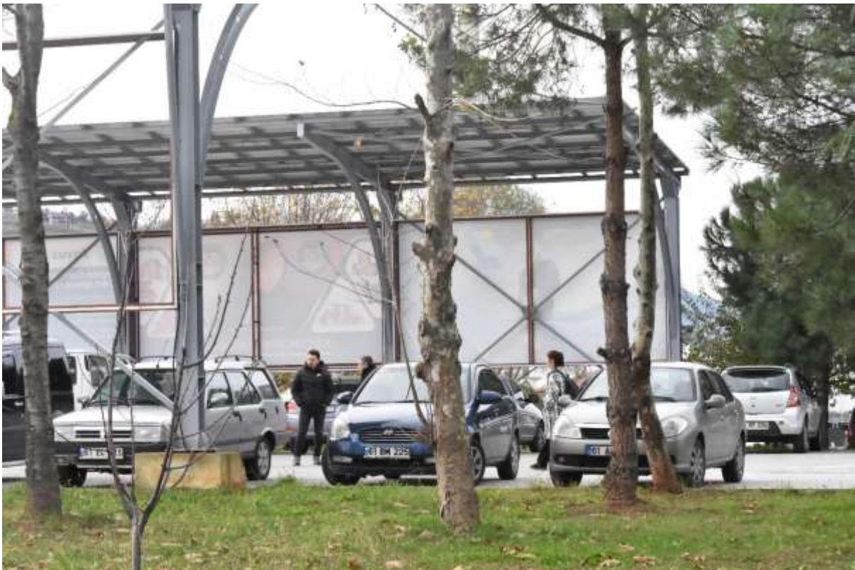
Photograph 23. General View of The Project Area
