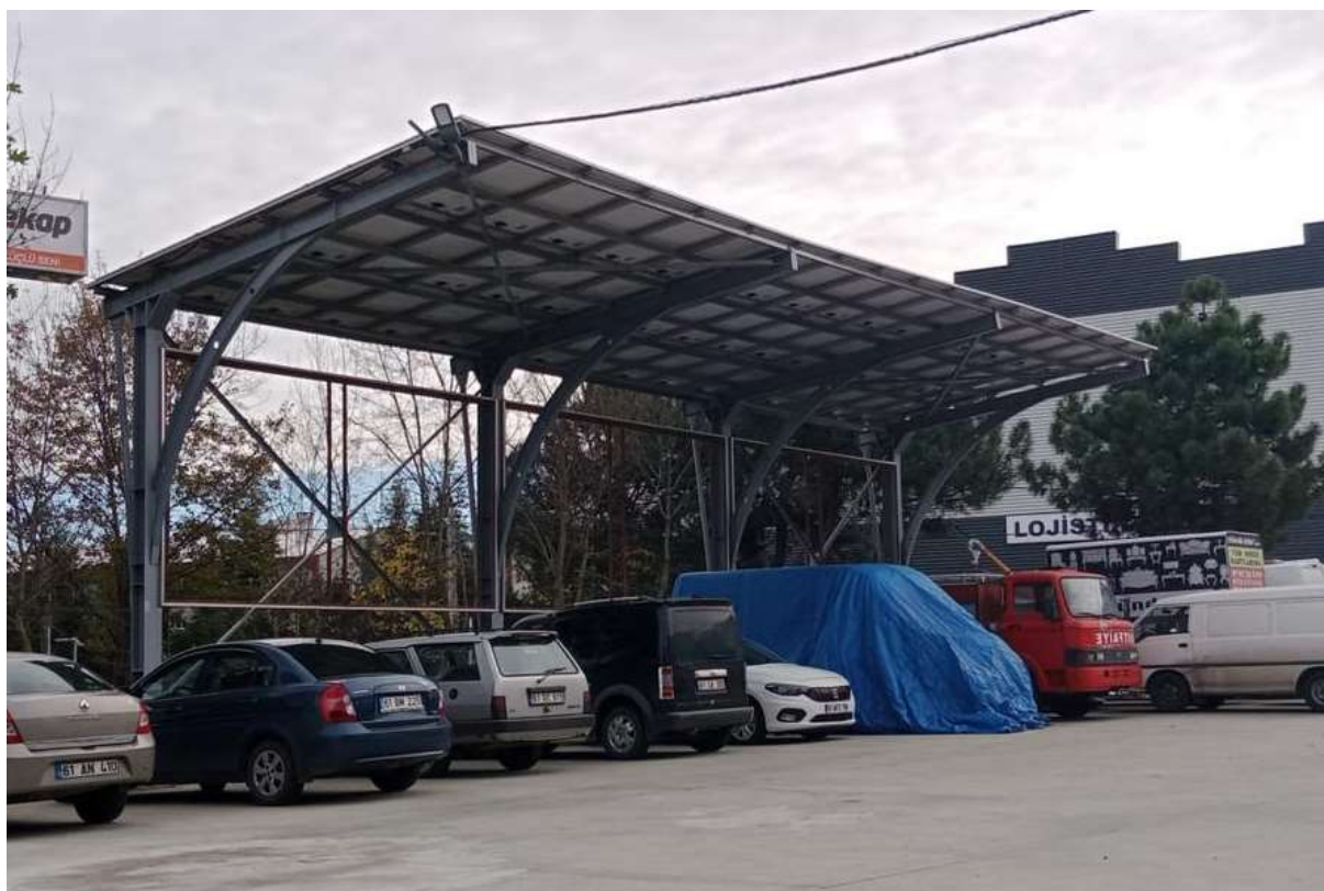
Photograph 1. Existing Carport Structure in the Project Area
