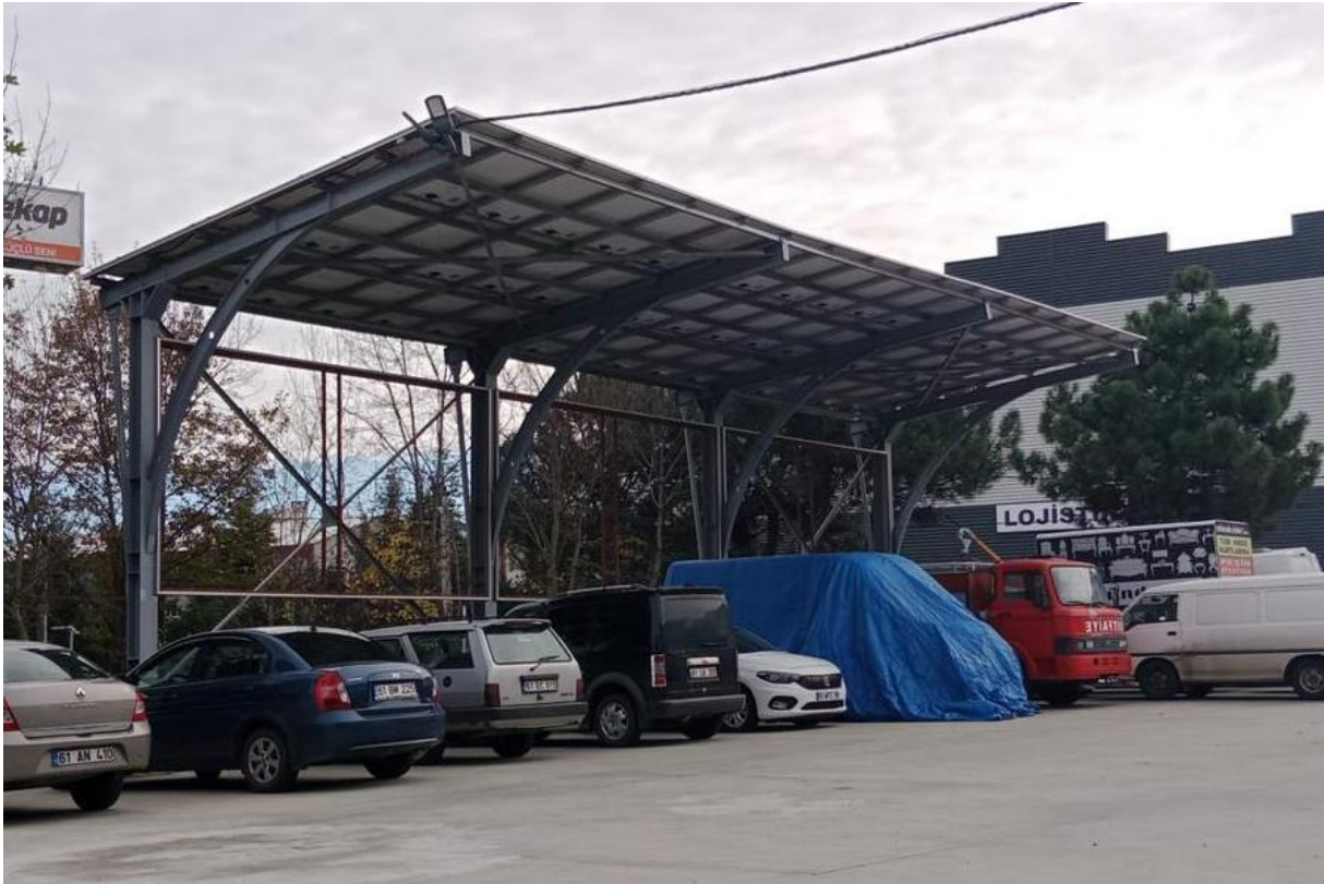
Photograph 1. Existing Carport Structure in the Project Area
