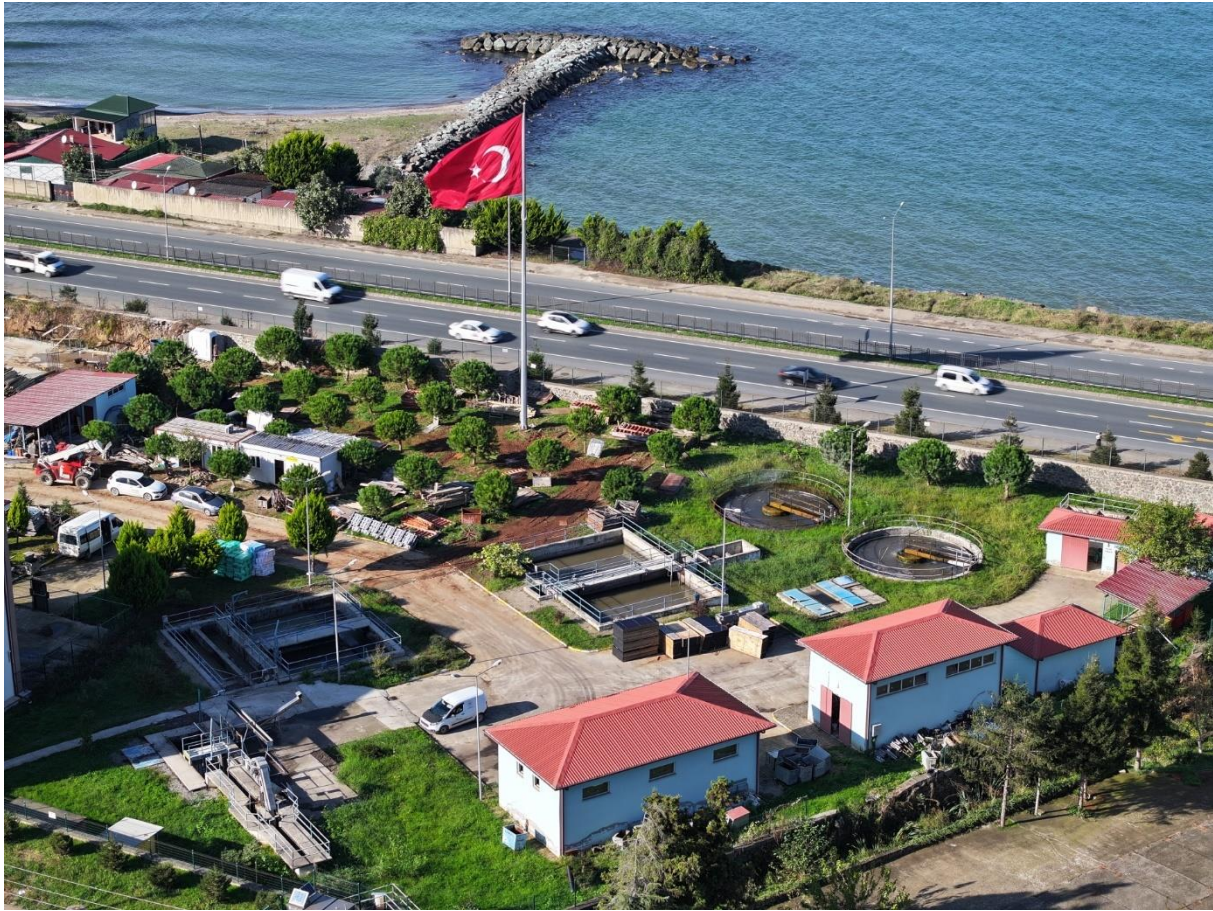
Photograph 11. General View of WWTP
