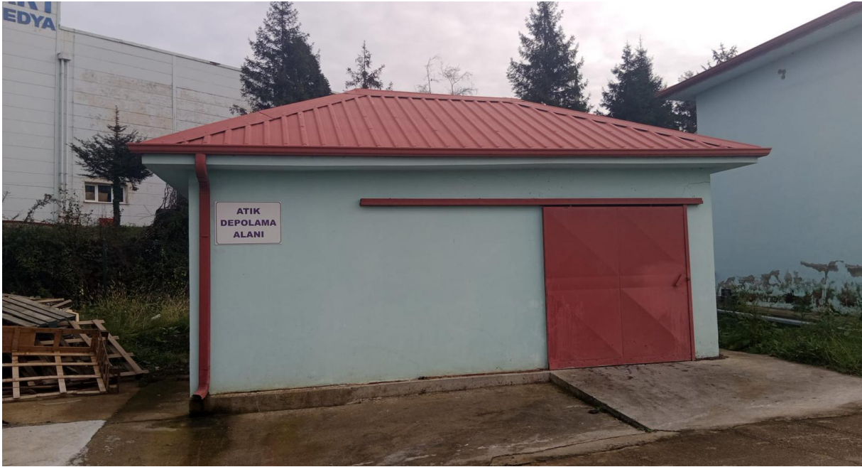
Photograph 18. Hazardous Waste Storage Area
