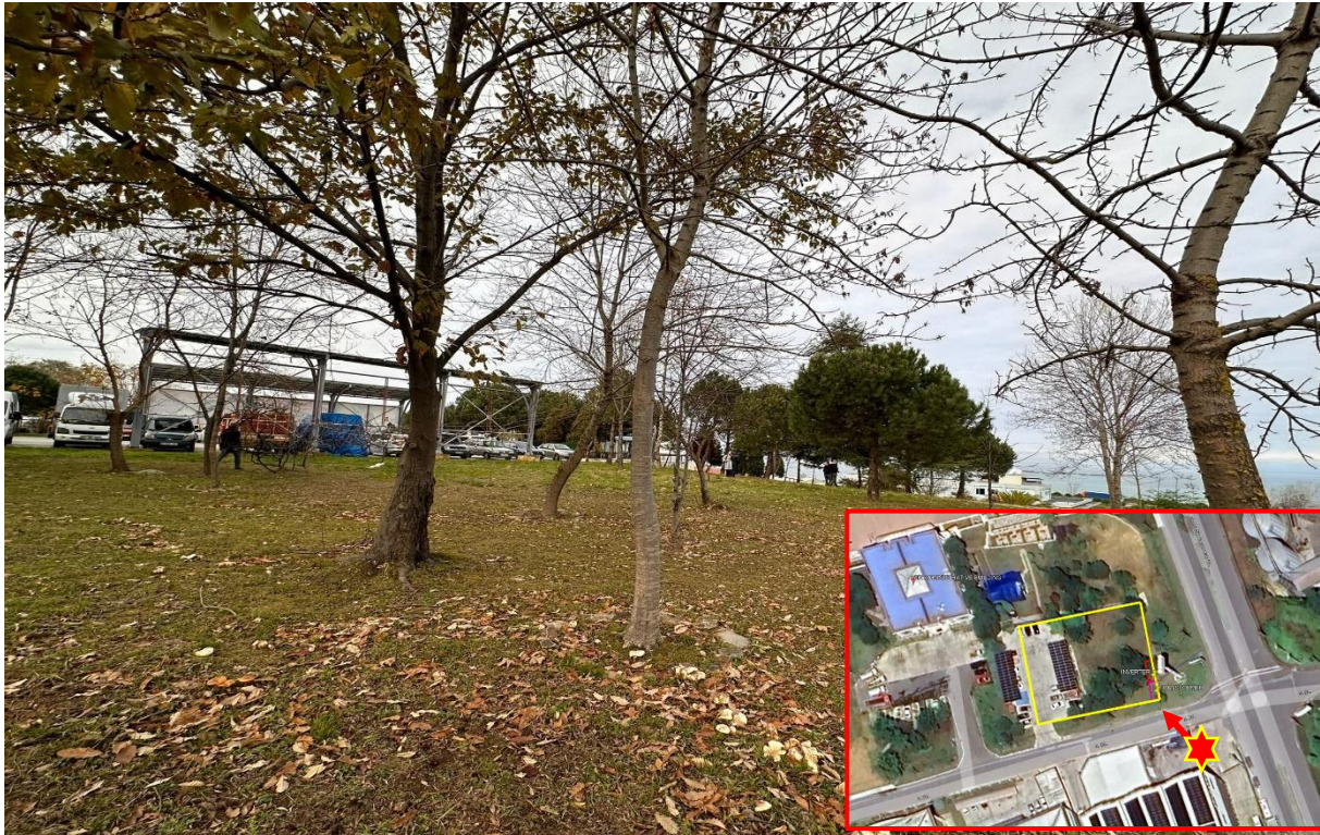
Photograph 6. View from Transformer Area
