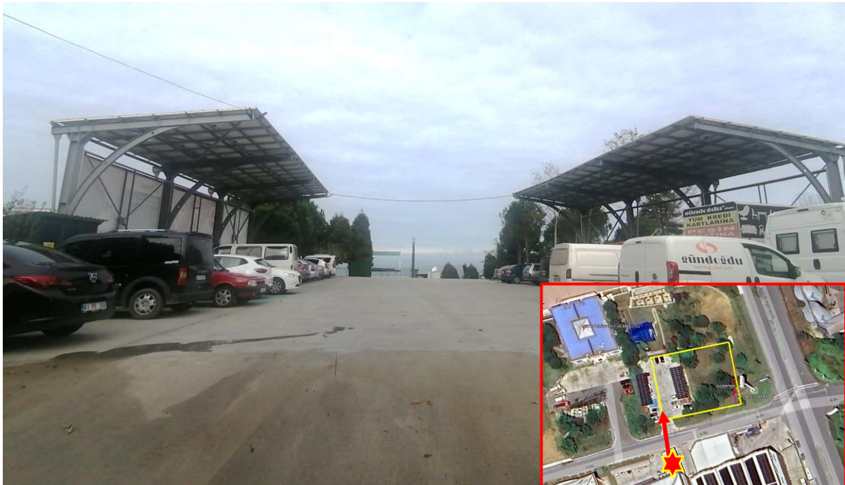
Photograph 3. Views from the Carport SPP Area-I
