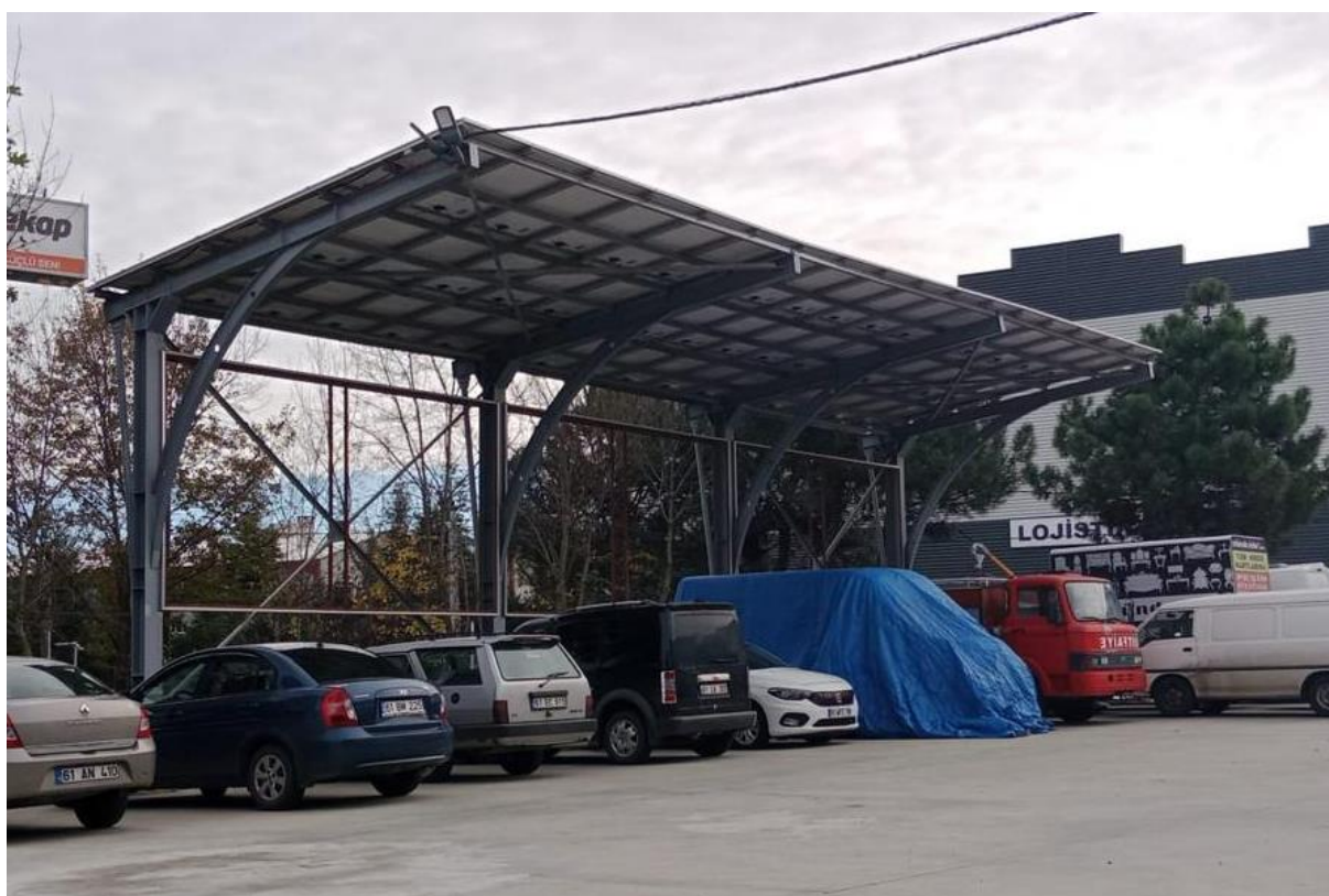
Photograph 1. Existing Carport Structure in the Project Area
