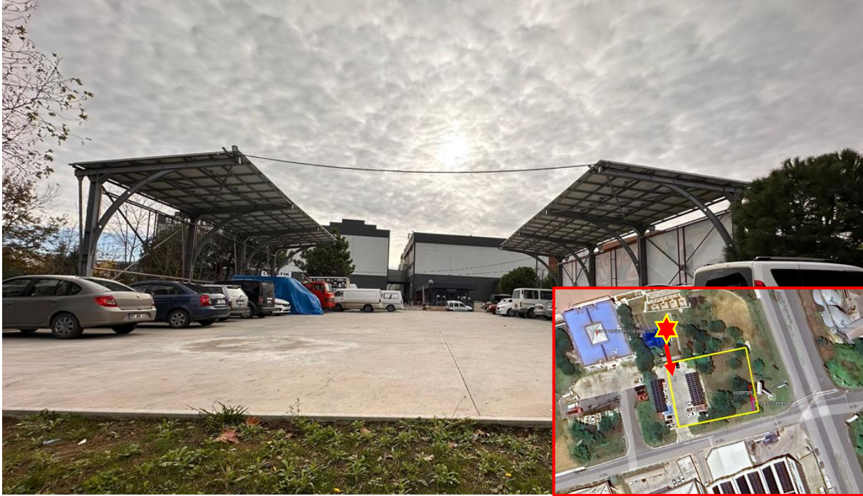
Photograph 4. Views from the Carport SPP Area-II
