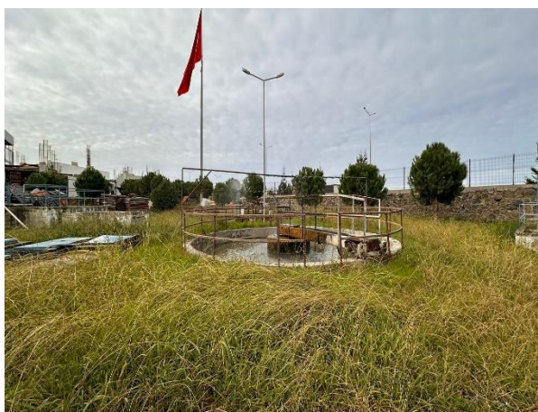
Photograph 14. Sedimentation Tank
