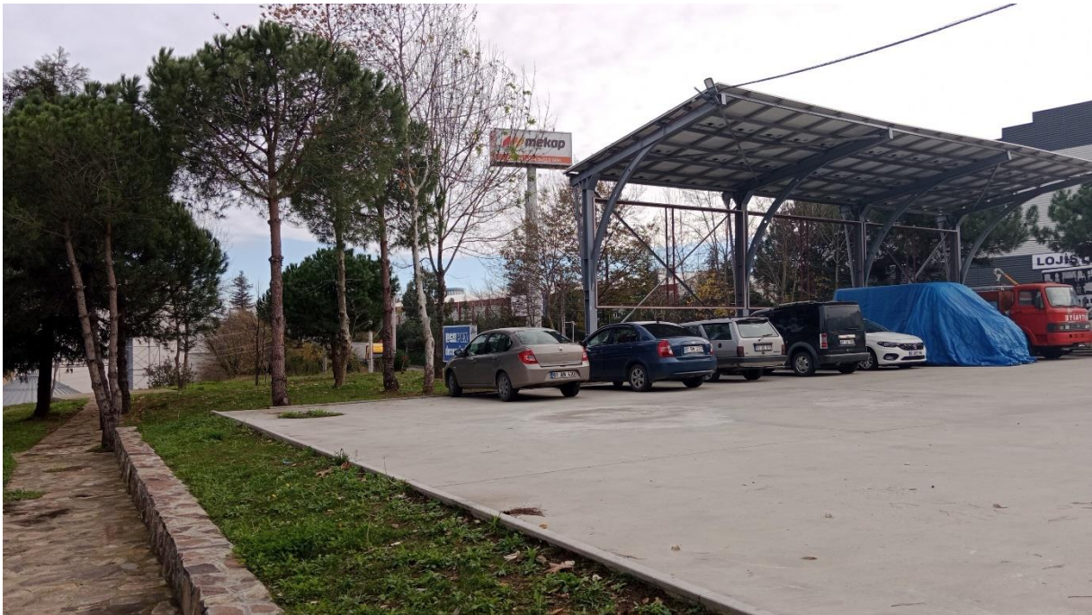
Photograph 25. General View of The Project Area
