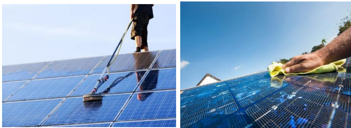
Figure 25. Illustrative Views of Panel Cleaning 39
