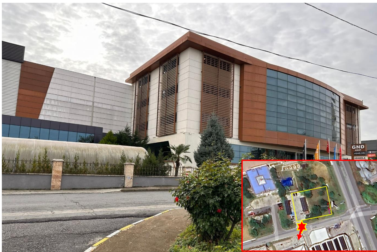
Photograph 10. View to the “Gündoğdu Mobilya” Office Building
